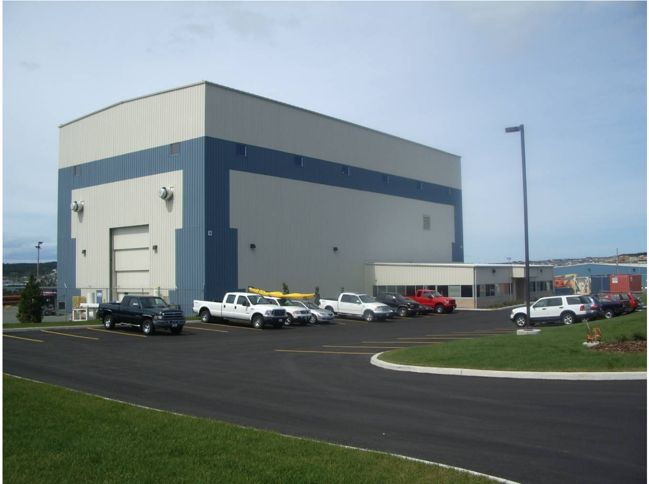
New Cameron Subsea Testing Facility in Donovan's Industrial Park
