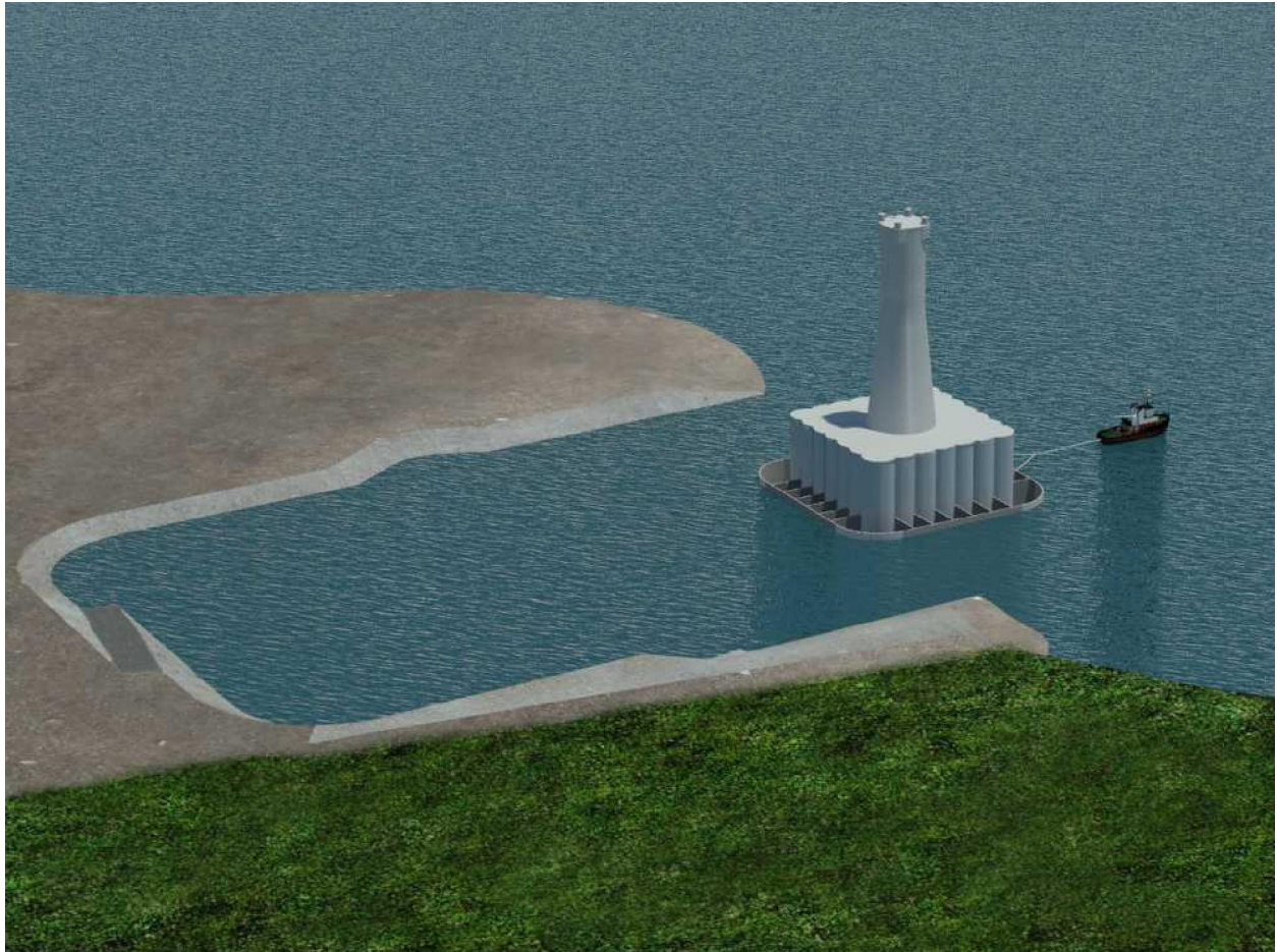
Figure 7: Float out of CGS from Graving Dock
